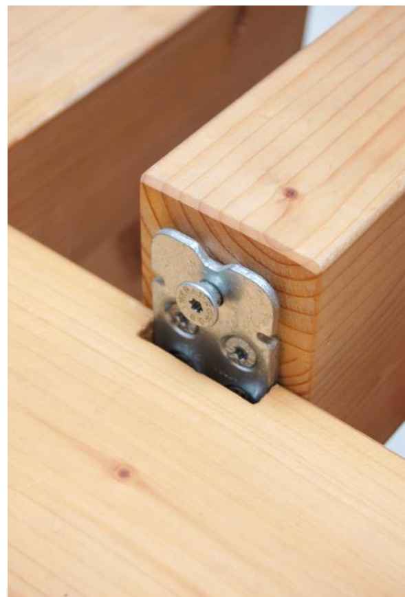
Typical concealed install
