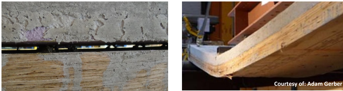
Fig. 18. Series 2 panel failure due to screw withdrawal (left) and timber tensile failure (right) - Brittle [5]
