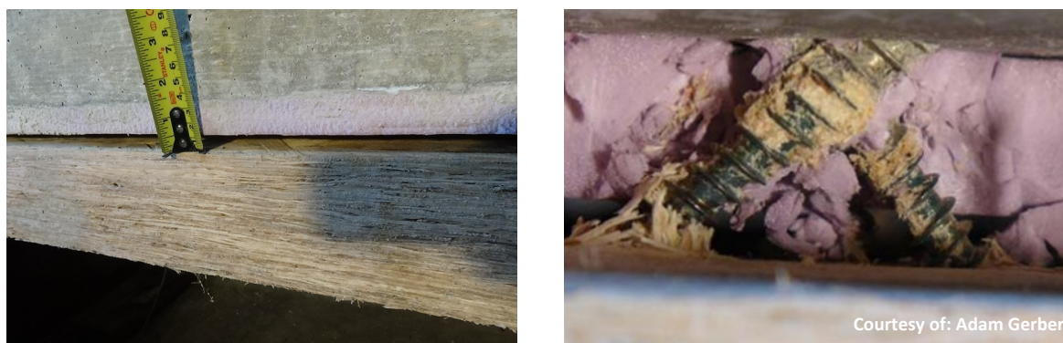
Fig. 20. Series 4 panel failure due screw withdrawal through 25mm of rigid insulation - Ductile [6]
