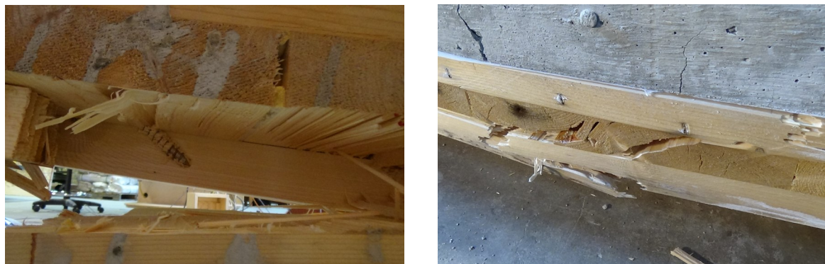
Fig. 19. Series 3 panel failure due timber tensile failure - Brittle [6]
