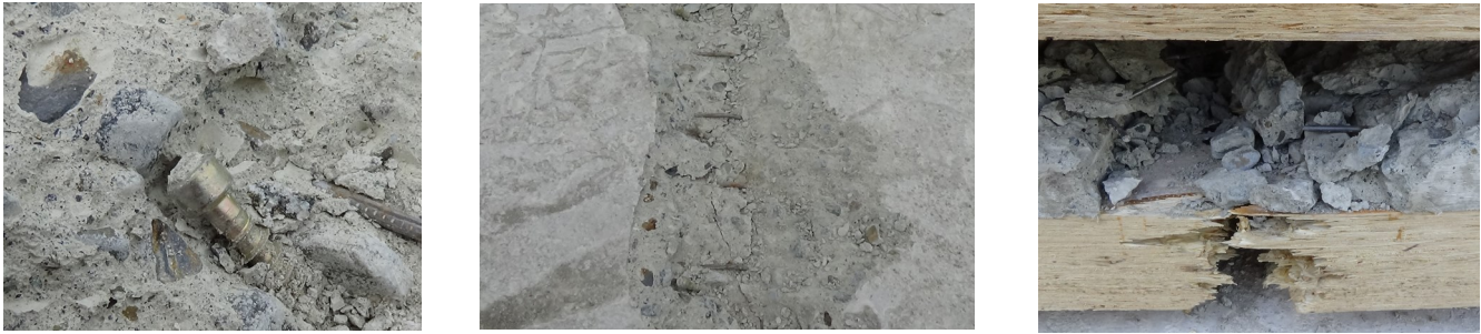
Fig. 17. Series 1 panel failure due to concrete crushing (left and centre) and timber tensile failure (right) - Brittle [6]
