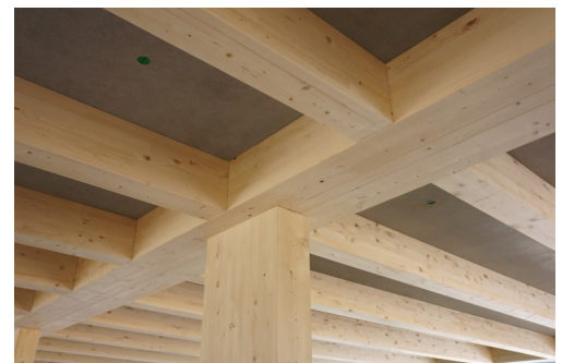
Fig.4– Interior view of office space with a TCC
