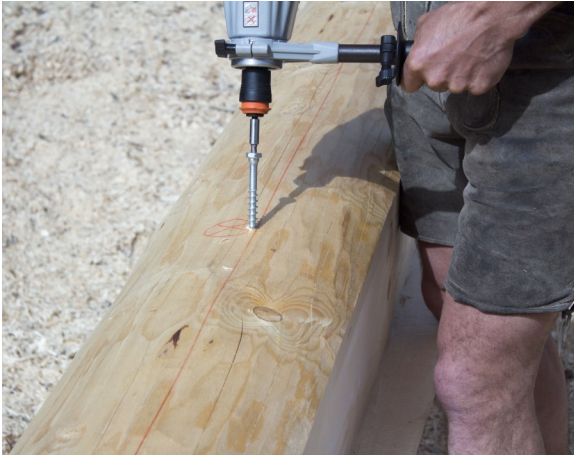
Install 1/2" x 6" anchor bolt
