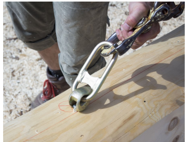
Engage lifting chains
