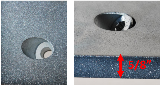
Typical machining requirement in steel plate to accommodate structural screw
