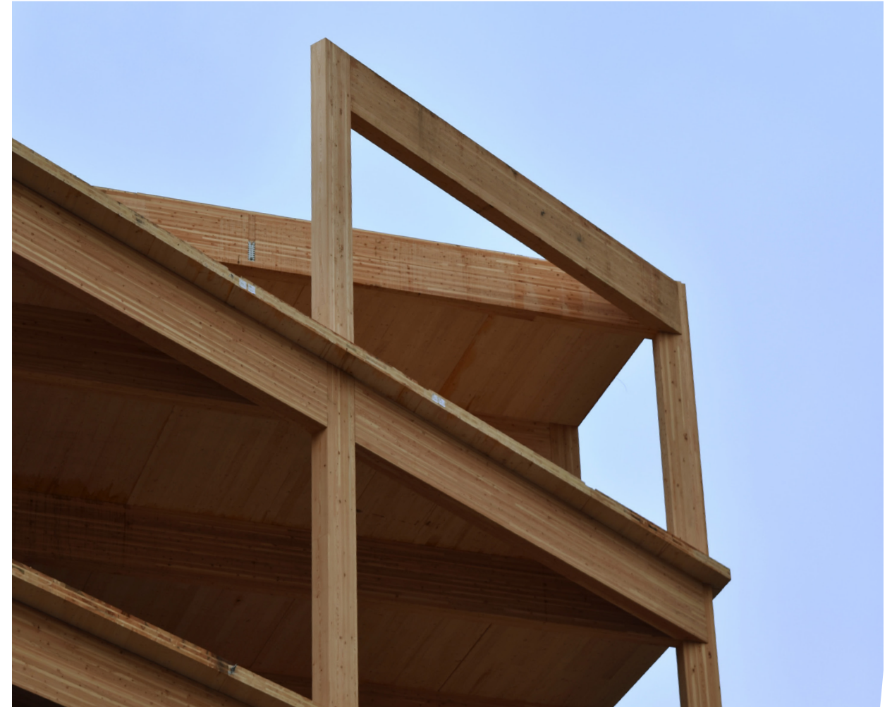
First Tech Credit Union Project in Hillsboro
