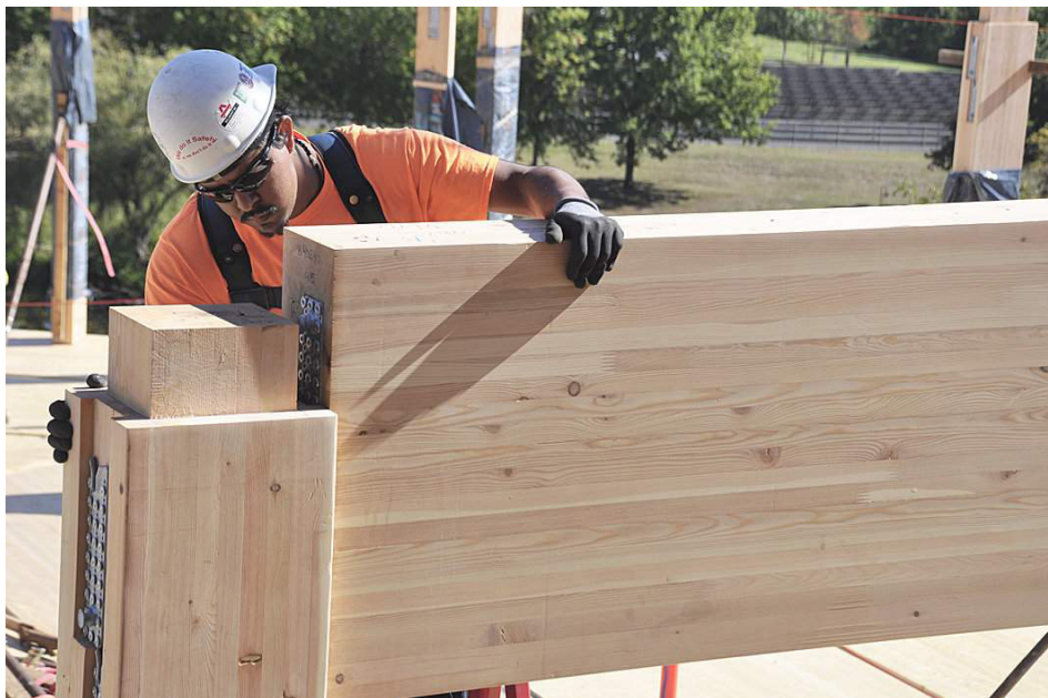
Install of pre manufactured Post to Beam connection First Tech building, Portland Oregon
