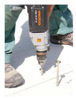
Screw installation at panel edge, for assembly purpose secures panel in place, fast
