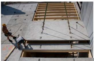
The pre-manufactured wood-concrete composite element is lifted into place. One crane lift per element.
