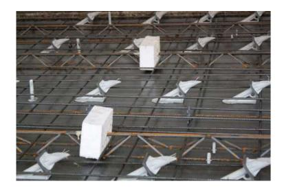
The concrete slab is entirely premanufactured in the concrete plant including required rebar, lifting anchors and ASSY® wood concrete composite connector.
