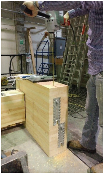
FIGURE 7, Installation of VG CYL reinforcing screw into beam member.
