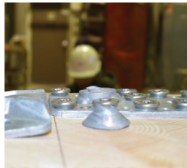
FIGURE 18, Breakage of collar bolt. Yielding of V-notch area on a connector also visible.
