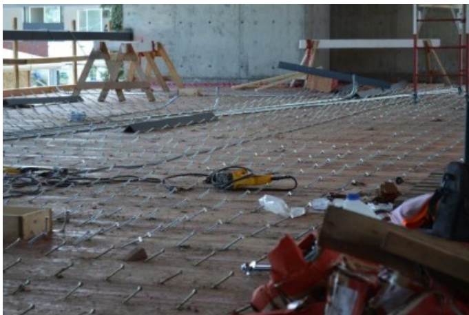
Figure 6: Project example TCC system utilizing STS @ 30° (photo credit Western Archrib—Structural Wood Systems)
