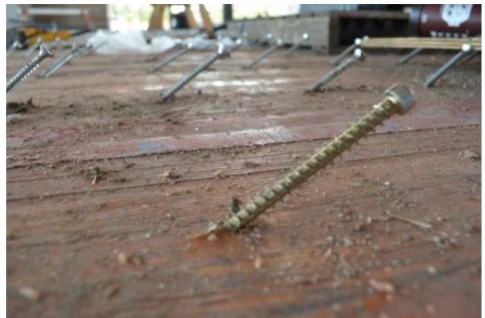
Figure 6: Project example TCC system utilizing STS @ 30° (photo credit Western Archrib—Structural Wood Systems)
